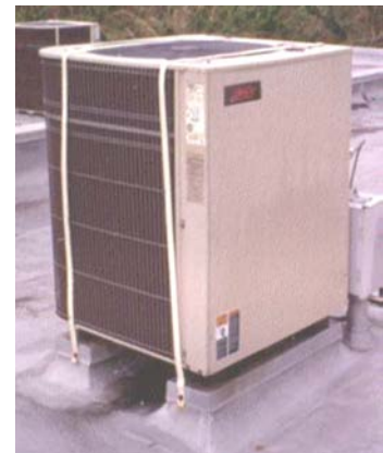
Better secured, two straps, 2 screws desirable per strap connection
