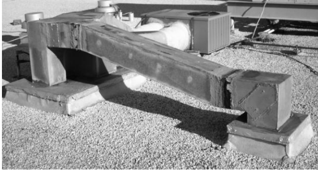
Exposed rooftop duct system
