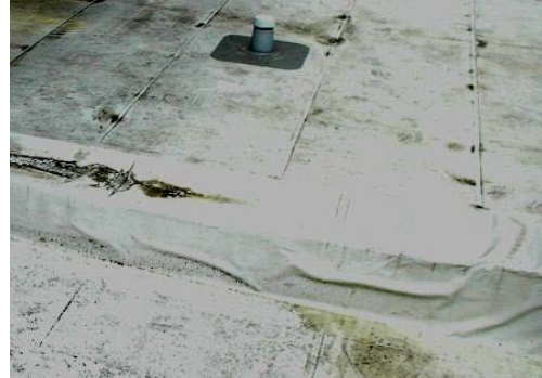
Duct system installed under roof cover
