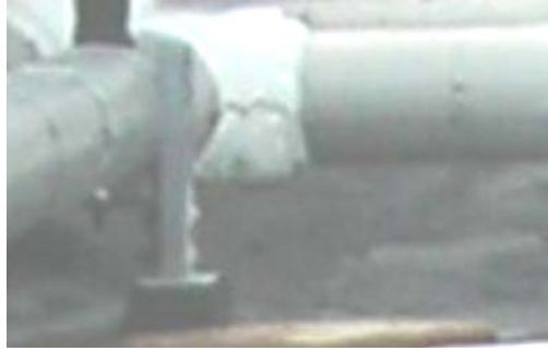
Pipe support on stands anchored to concrete deck
