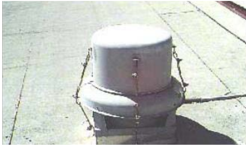
Fan and cowling secured with wire rope
