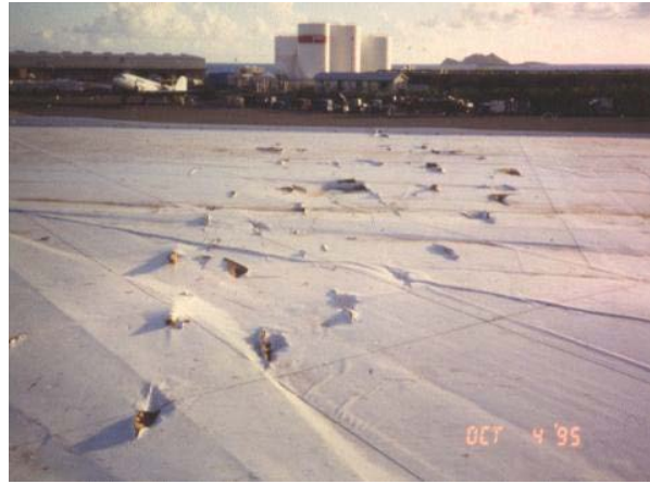
Roof cover damage from rooftop equipment
