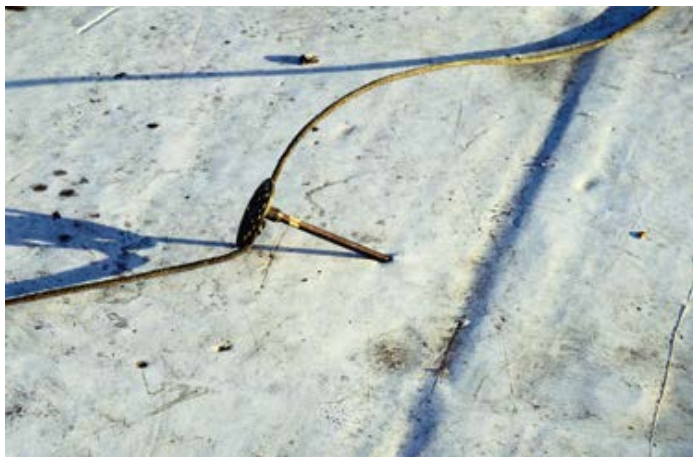
Air terminal penetrating roof cover
