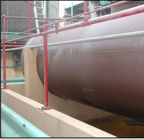
Outside main fuel tank secured against buoyancy by wrap-around concrete saddle
