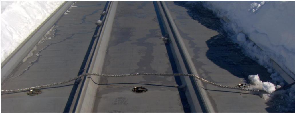
*Lightning protection cable (Photo source: Zurich)*
